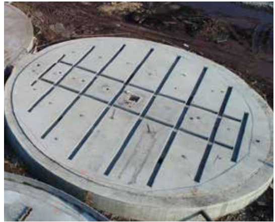
— Photo of floor aeration channels cast into concrete
