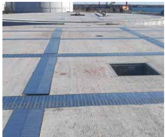
— Photo of floor aeration with grids mounted
