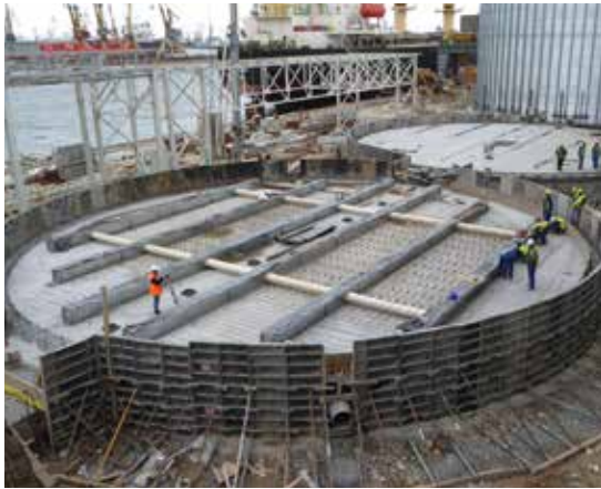
— Photo of aeration channel civil works
