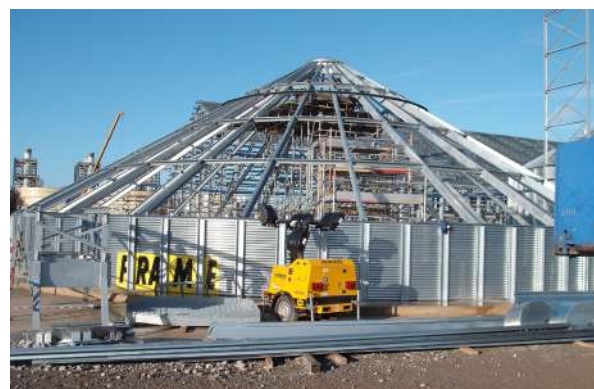
— General views of the FRAME roof.
