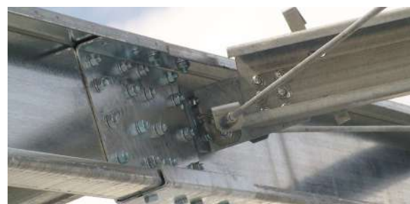
— Intersection of tie bars & purlins
