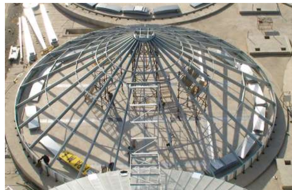
— Internal roof structures
