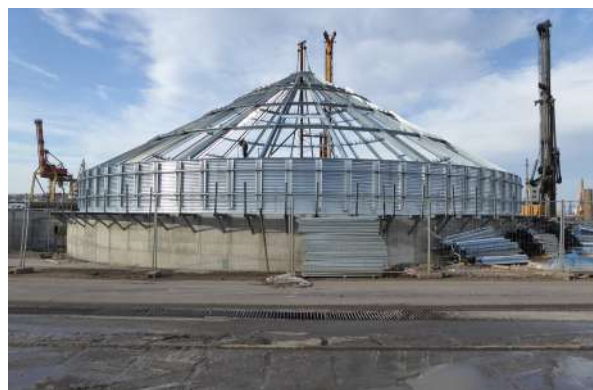
— Roof and Roof Structure
